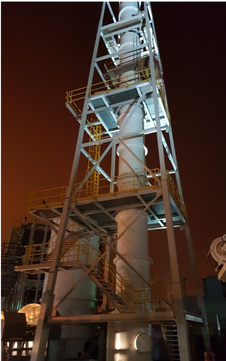
Stack Pipe and Structure assembly and erection
