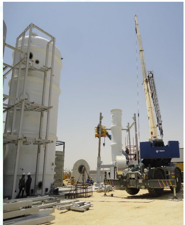
Scrubber Tank and Structure Assembly and Erection
