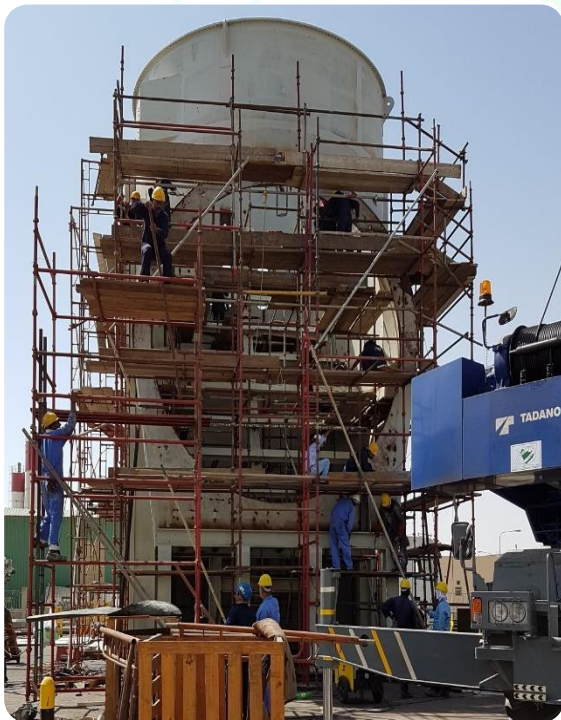
After Burner/Secondary Combusting Chamber fabrication
