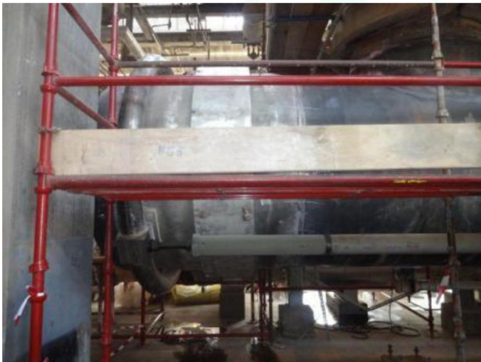
▲ Replacement of Expansion Below Gimbaled Joint 42"Ø HC Line SS Pipeline. (4 th Floor)
