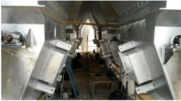
Erection of Hooper's
