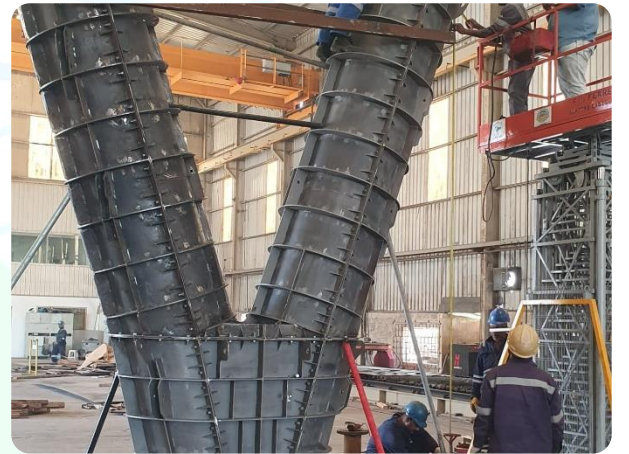
Shuttering Pier "Y" Shape
